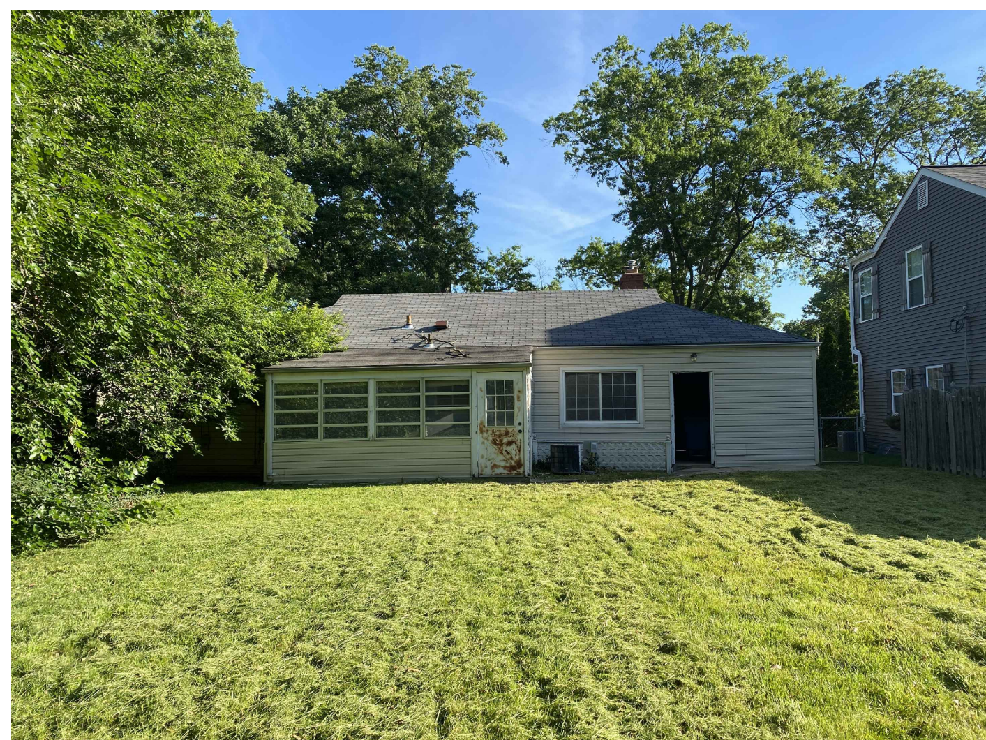
814 alexandra avenue - existing rear
