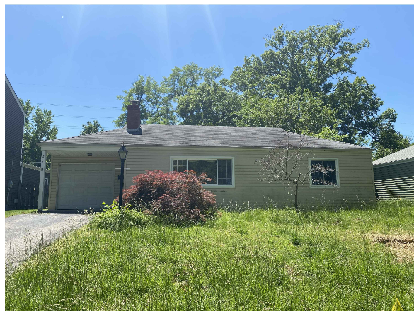
814 alexandra avenue - existing front
